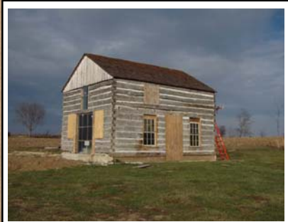
Cabin Under Restoration in 2012 and 2013 Photo: Terry Hannan
