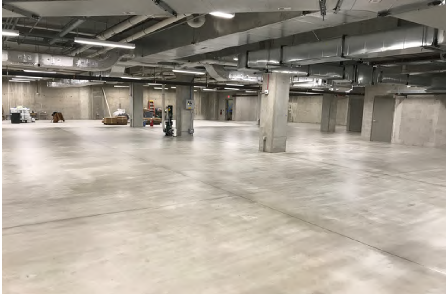
Basement Floor Sealer & Cleaning
