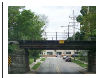
UPRR Rail Bridge on Pearl St. in DeKalb
